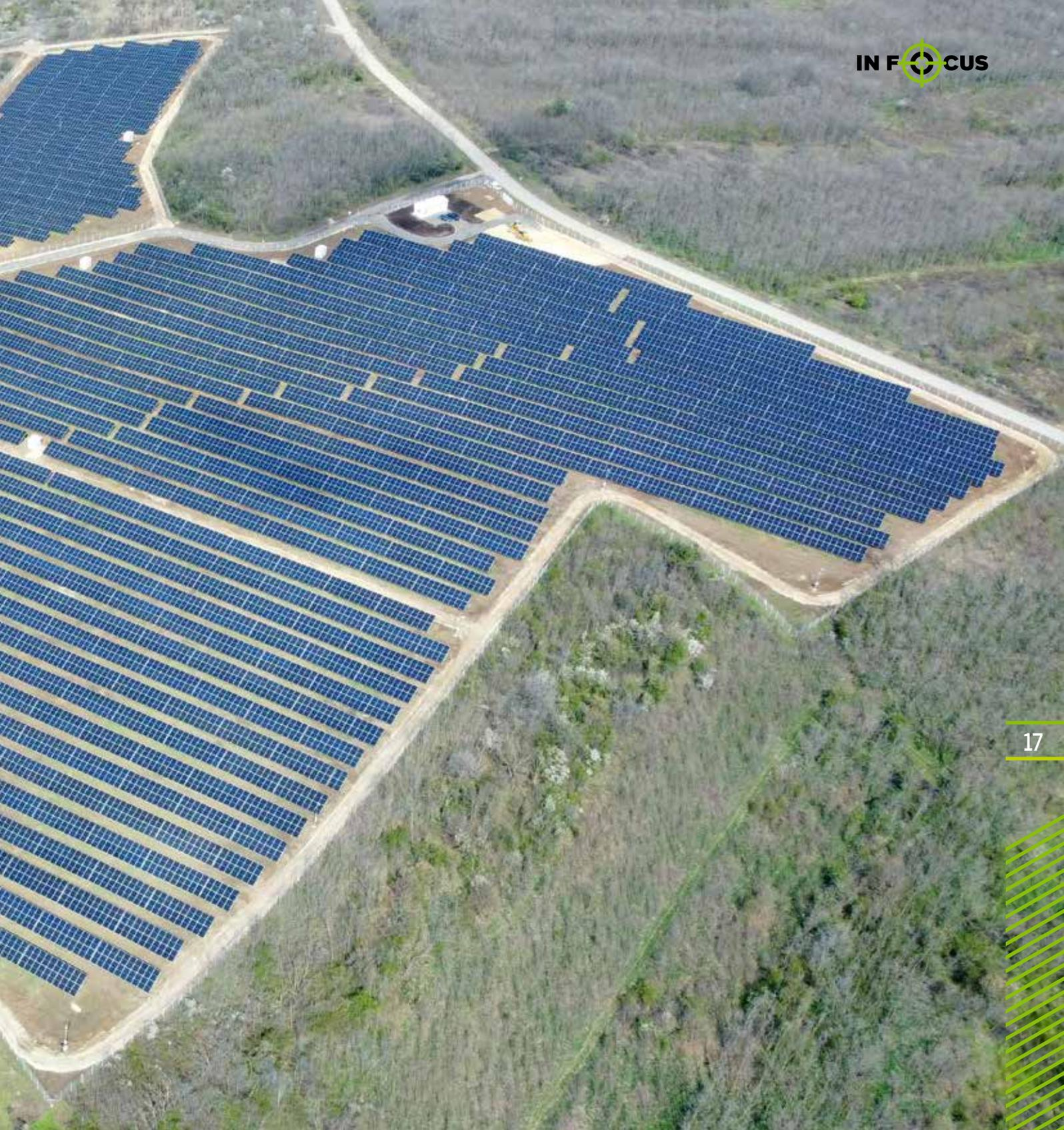
Bifacial solar panels were used to construct this solar power plant, which can yield electricity from both sides of the panel, which is why they generate a larger amount of electricity. The solar panels are placed on a specially-made construction that allows greater absorption of reflected radiation.
