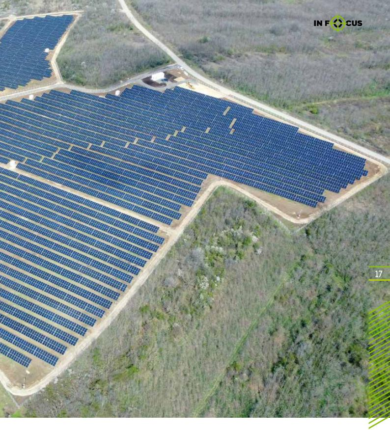
Bifacial solar panels were used to construct this solar power plant, which can yield electricity from both sides of the panel, which is why they generate a larger amount of electricity. The solar panels are placed on a specially-made construction that allows greater absorption of reflected radiation.
