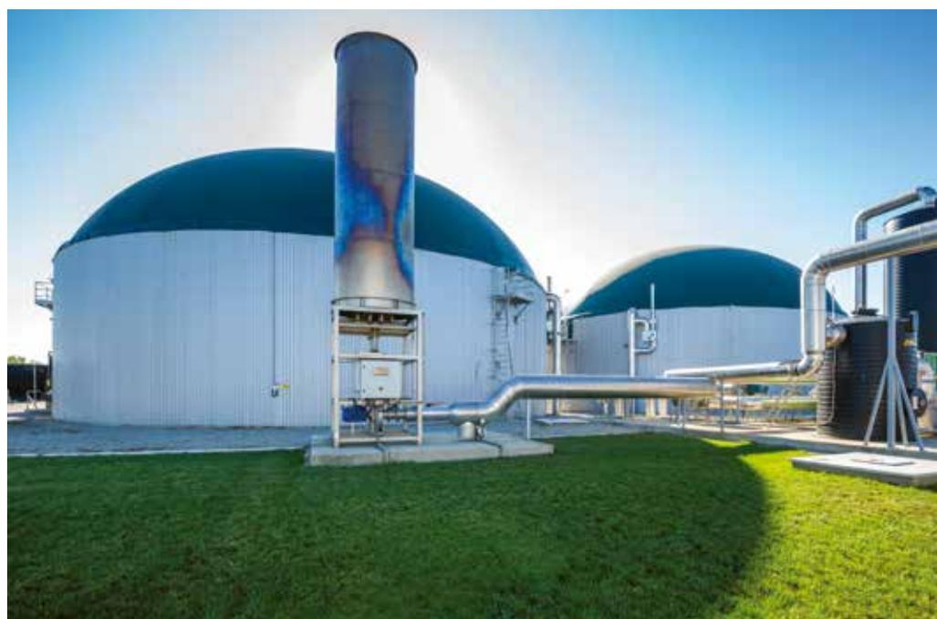
acetogenesis and methanogenesis, a considerable amount of gas with a high percentage of methane (40-65 per cent by volume) is produced, which is called biogas (medium thermal power 16.2 - 19.8 MJ/Nm<sup>3</sup>).
